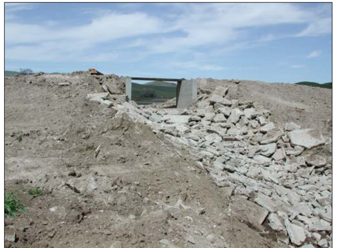
The overflow structure in which headboards can raise or lower the depth of the upper wetland
